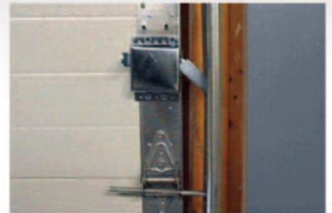
Traditional lock under pressure fails
